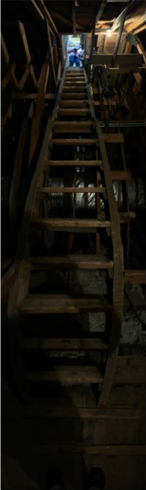
Rock Church Clock Tower Ladder
