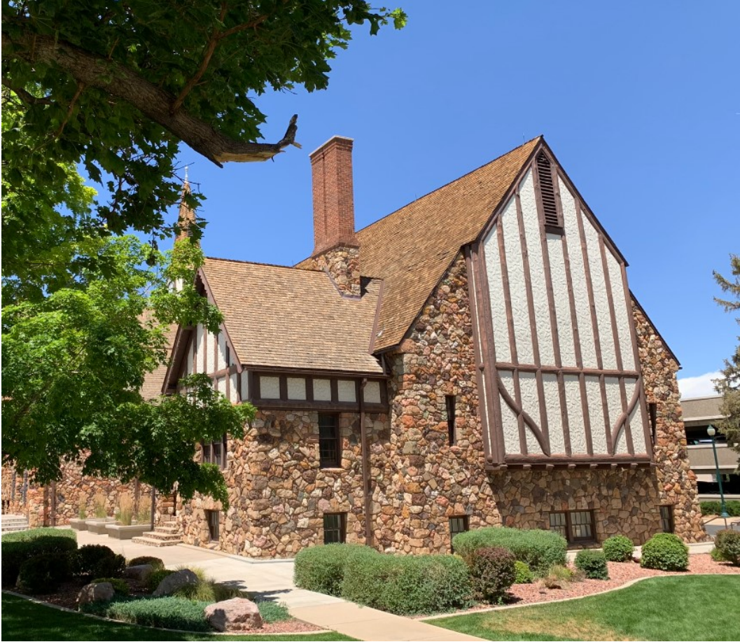
East Side of Rock Church
