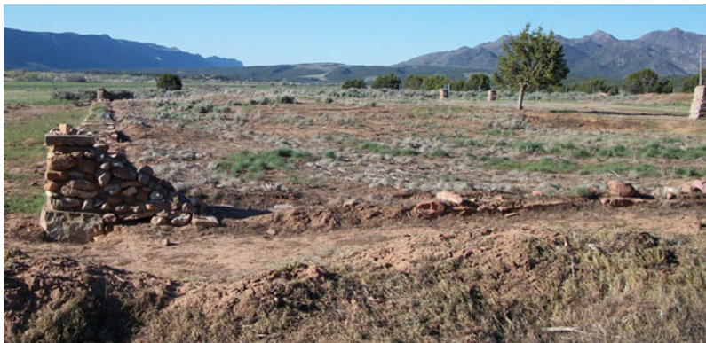
Fort Harmony foundation from north east corner.
