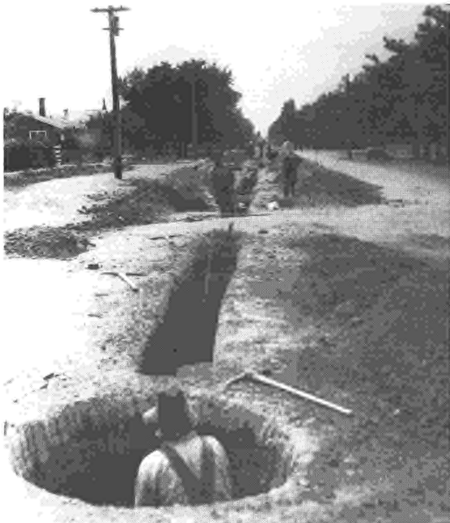
"Hand Digging Sewer Trenches" Public Works Administration Project (W.P.A.) During 'The Depression' 200 East and 200 North, looking west--1934
