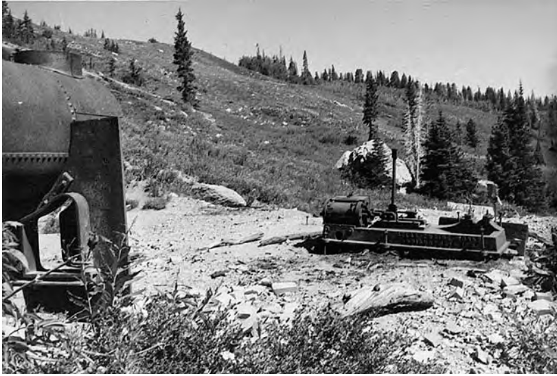
The remains of steam hoisting equipment and a boiler at Baby McKee inclined shaft in Cardiff Fork in Big Cottonwood Canyon reveal changes in mining technology. Built by Atlas Engineering Works in Indianapolis, this equipment was installed in the 1890s or early 1900s. The nearby Monte Cristo prospecting shaft (not shown), sunk during the 1917 silver boom, featured an electrically powered hoist. Photo by L. P. James (1974).
