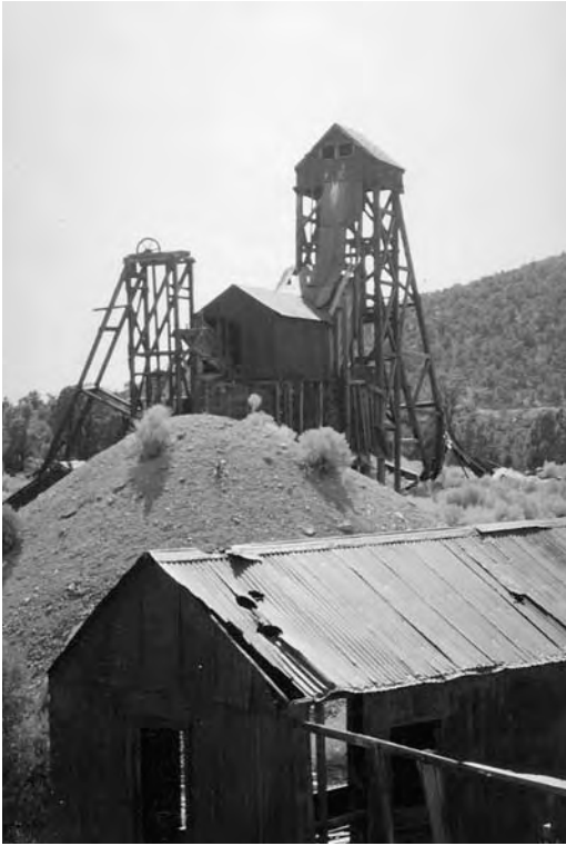
Frame scaffolding remained in 1996 at the Jennie Mine in the Gold Springs District on the Utah/Nevada border. Photo by Janet Seegmiller.
