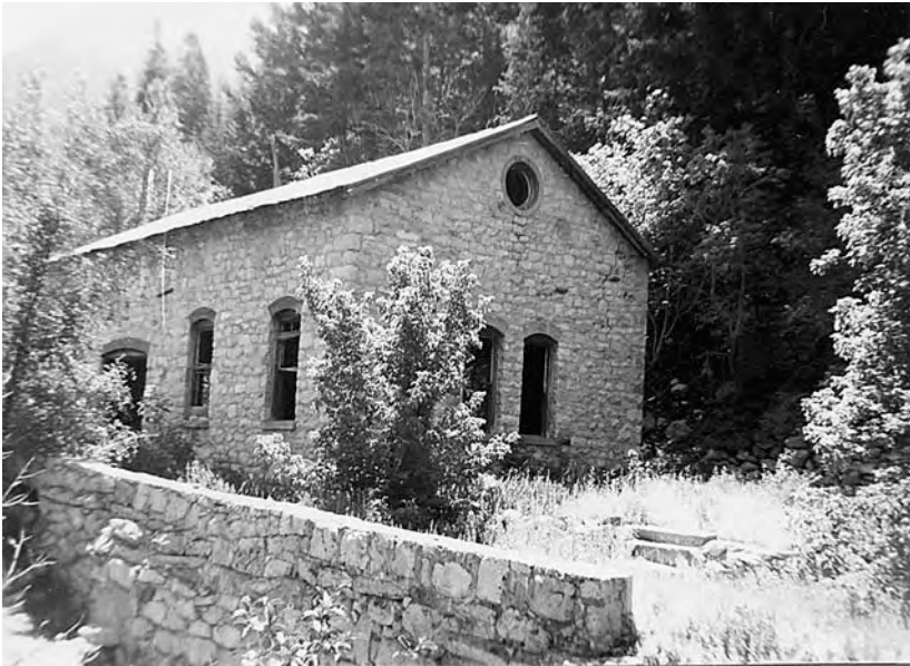
Ruins of the Wasatch Power Company plant stand below Tanners Flat in Little Cottonwood Canyon. Installed in 1904 by Columbus Consolidated Mining Company, two water-powered turbines generated electricity for the air compressors, mills, and miners' dwellings at Alta. Photo by L. P. James (1963).
