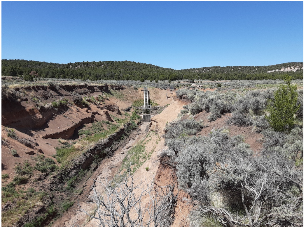
The trench to the tunnel that goes from Grass Valley to Pinto Creek on the other side of the ridge, was one of the first diversions of water from the Colorado River drainage to the Great Basin. Jay Jones photo.
